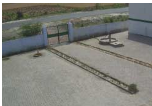
Paving of the School ground
