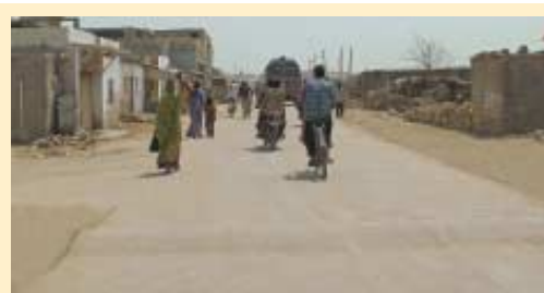
The new all weather cement concrete road at Surajkaradi.
