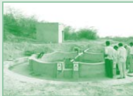
WASMO Comm. Well & Pump House at Khatumba
