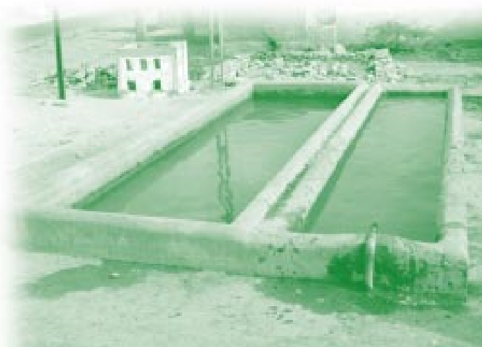
Infrastructure cattle trough at Padli
