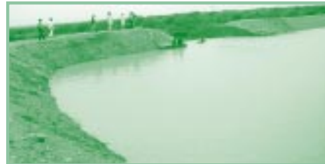
WSM Ambaram dam of village Vasai, under DRDA watershed development project
