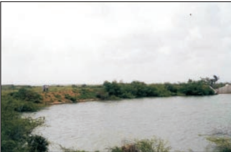
Dam after rains
