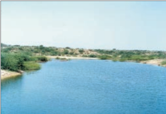
Dam at Tupni village after rains
