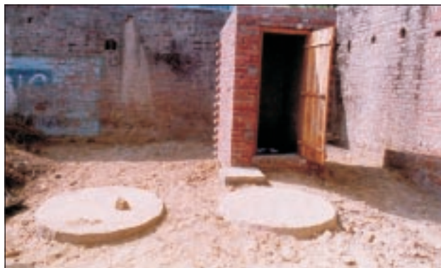
Low cost latrine
