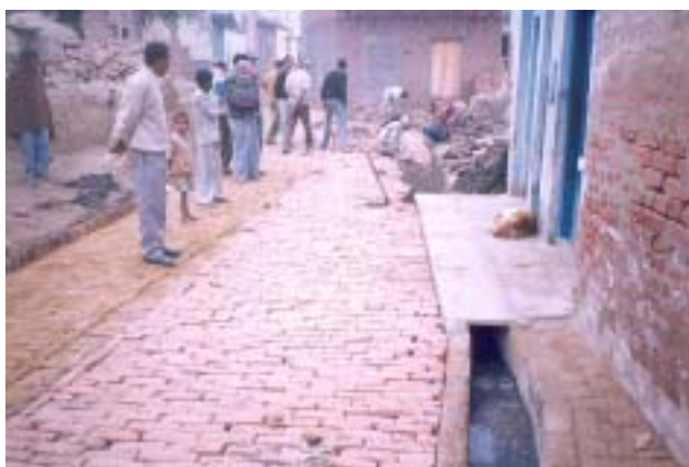
Construction of brick paved tracks
