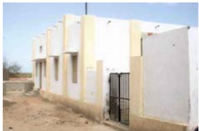
Aganwadi building repaired
