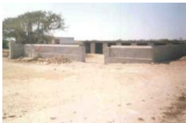
Cattle shed constructed as a part of entry point activity.
