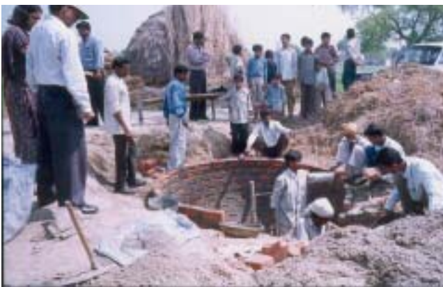
Construction of Bio-gas Plant in progress
