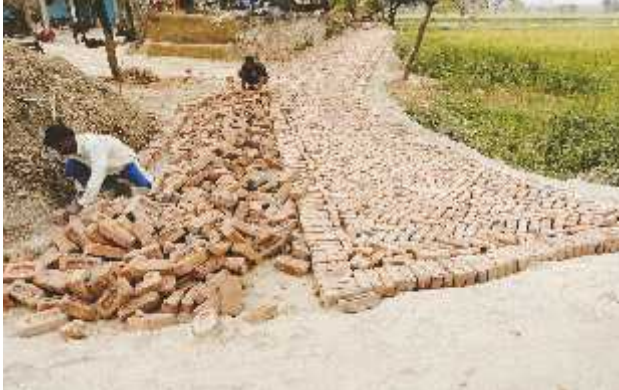
Brick pavement repair work
