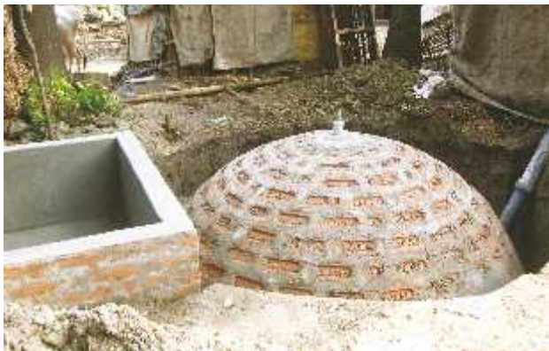
Bio Gas Plant - Deenbandhu Model
