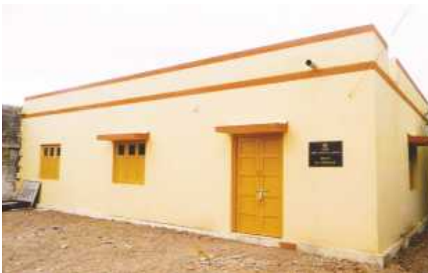
Completed work SNTD classes building, toilet block
