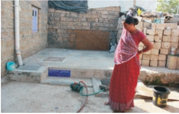
Roof rain water harvesting
