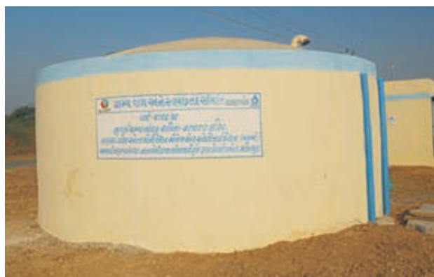
Drinking Water tank
