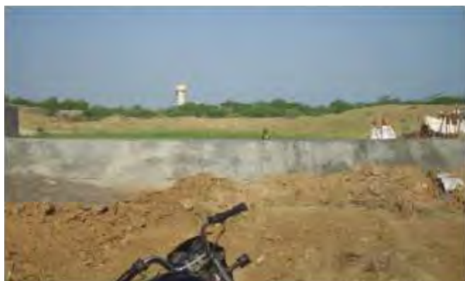
Kuthkabadi Check dam
