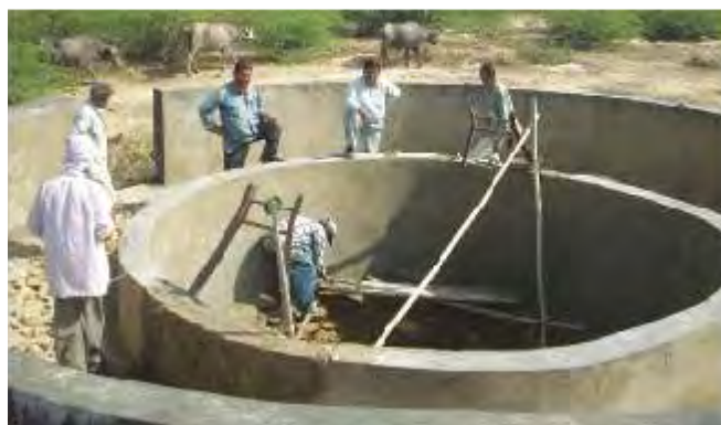
Community well construction in progress
