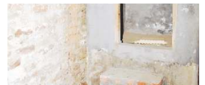
Construction of Toilets
