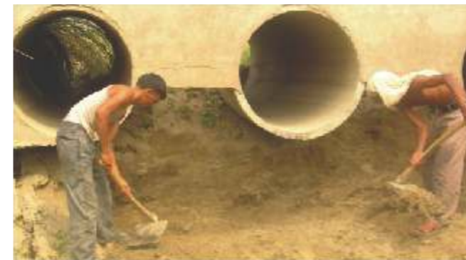
Culvert construction in progress
