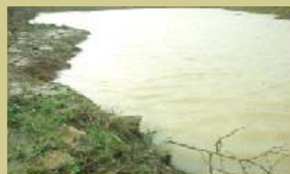
Sanvalo dam filled up during monsoon
