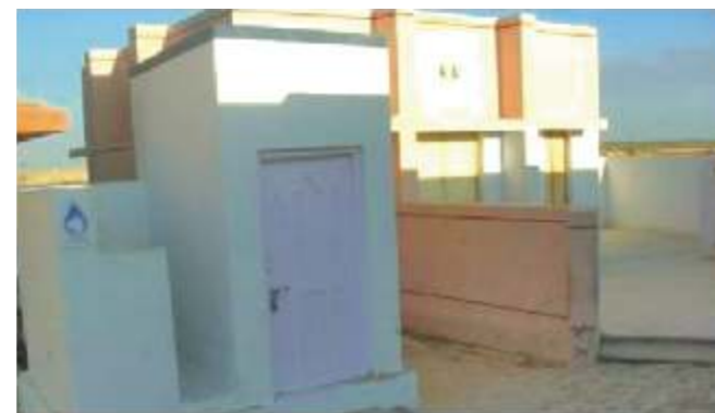
Sanitation unit at school
