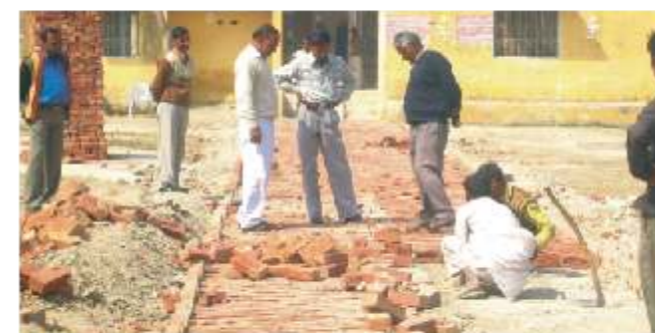
Brick paved tracks construction
