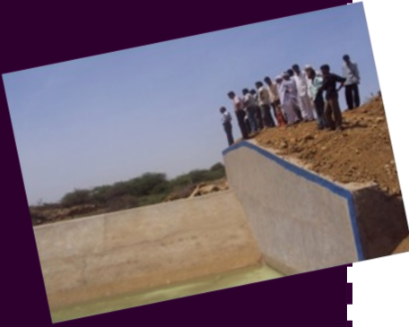
Check dam at Gurgadh.
